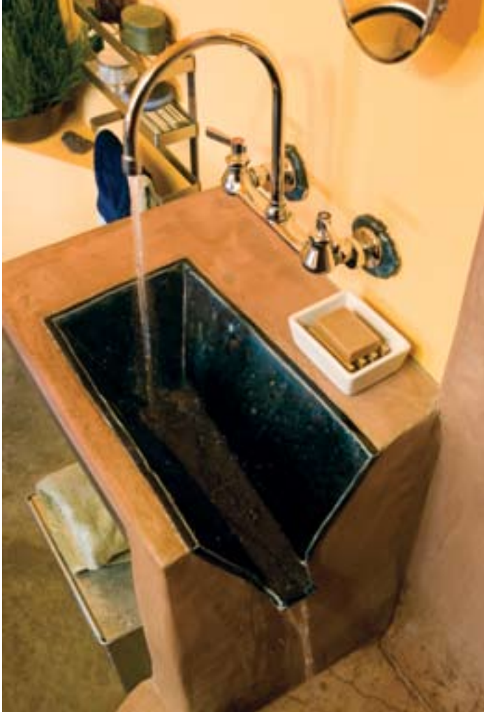
The three-sided sink drains into the shower, eliminating the need for a second drain. The shower drains to a graywater system, which irrigates the yard.
